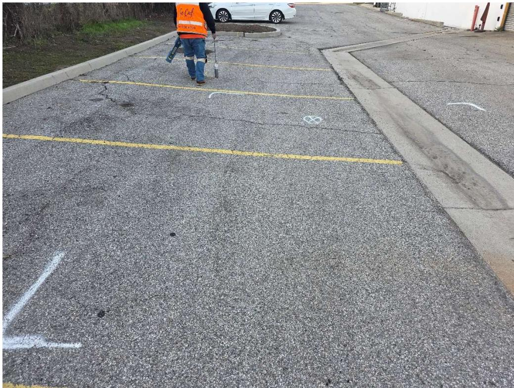
**Photo 1** View of geophysical survey being performed in the vicinity of a marked boring location.
