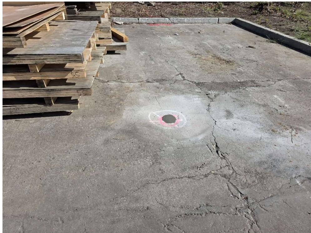
**Photo 7** Photo of completed concrete patching at boring location.
