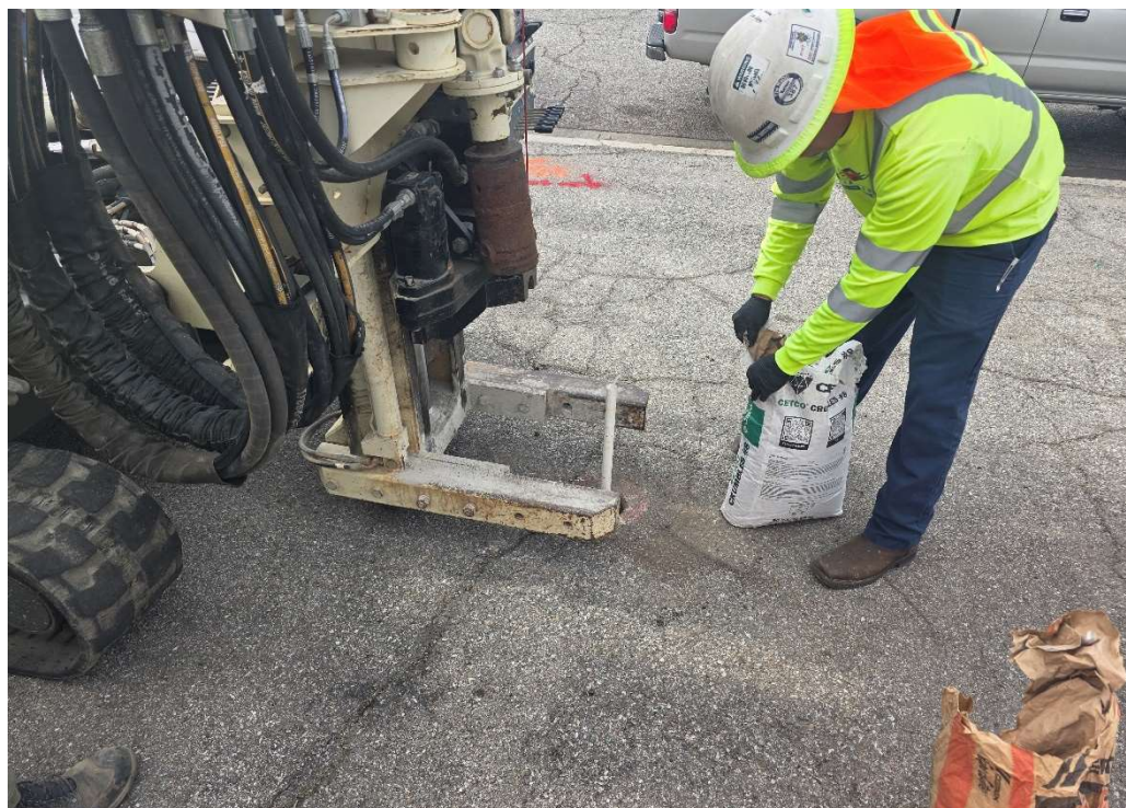
Photo 4 View of soil gas probe installation at location SGP-1.
