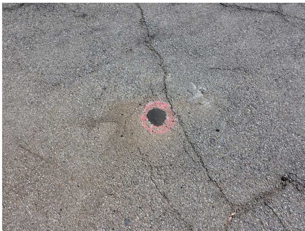
Photo 6 View of SGP-1 patch after soil gas sampling.
