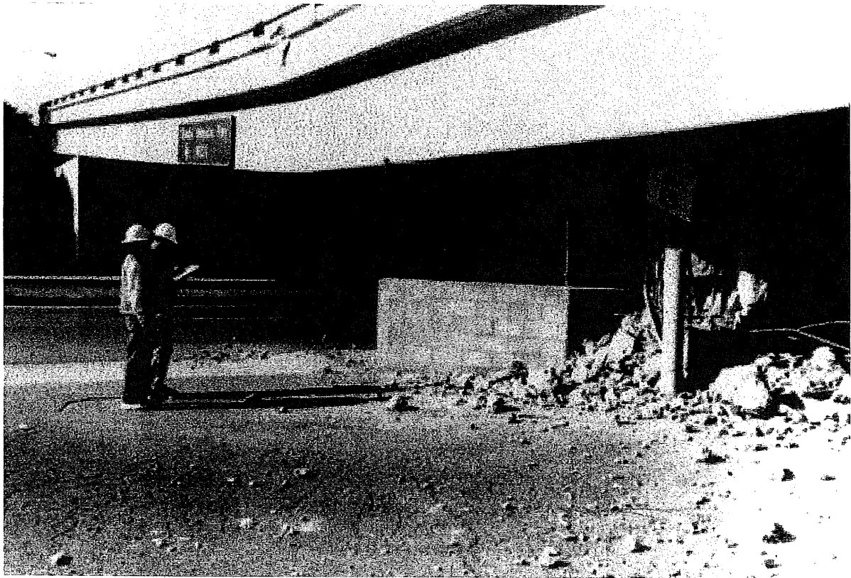
Santa Monica Freeway (I10) Collapsed Overpass 1994 earthquake
